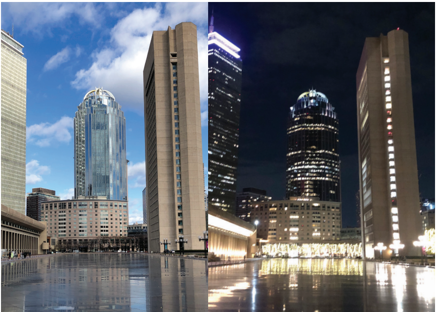
Fig 13: Photos of 111 Huntington Avenue, a Boston skyscraper, 2022
